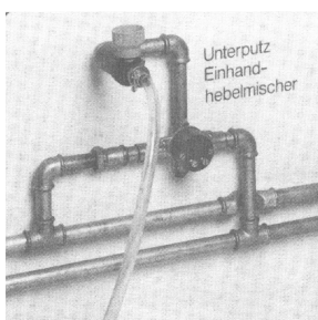
Typical Installation: Flushing of single lever mixers.
